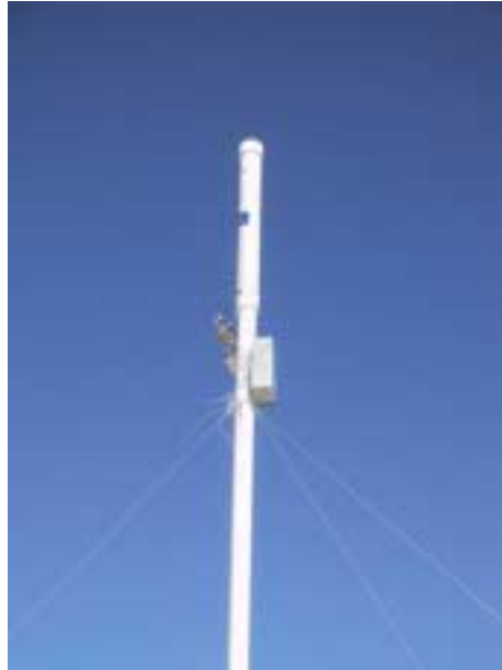
Figure 2a. Installed “Backpacker” 20-Meter Test Antenna (Radome Installed)
