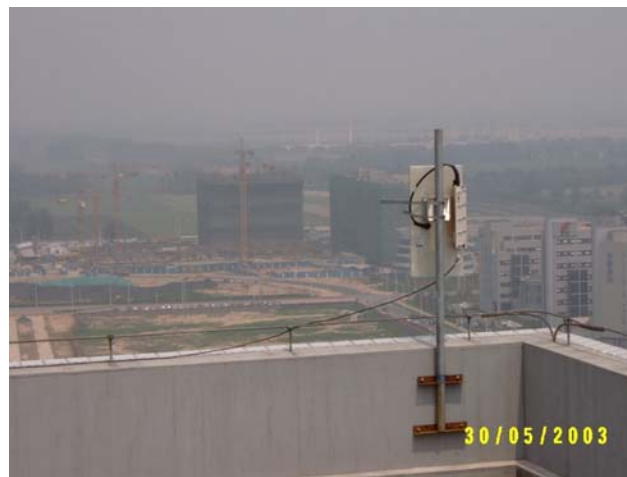
Figure 9: Beijing - View from the base station building
