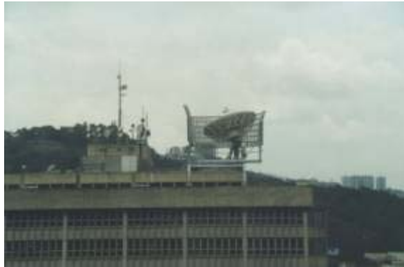
Figure 29. Mesh screening acting as interference shielding in Caracas
