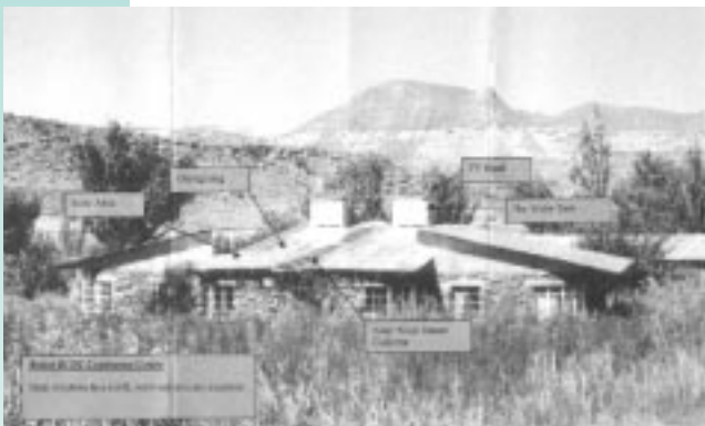
Figure 6.11. Main conference center showing RE applications.
